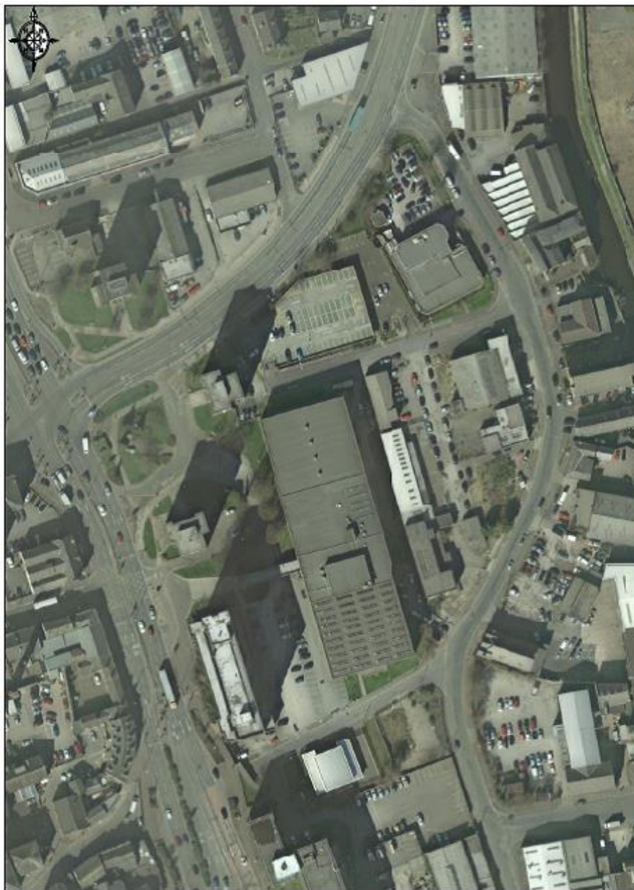
Figure 3. Aerial view pre-demolition
